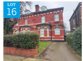
Flats 1–5, 7 St. Edmonds Road, Bootle, Merseyside L20 7AJ
