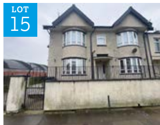
Flats B and C, 443 Stanley Road, Bootle, L20 5DN
